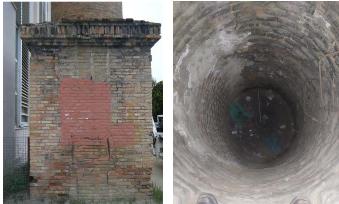
Figures 5 i 6. Exterior e interior base xemeneia
