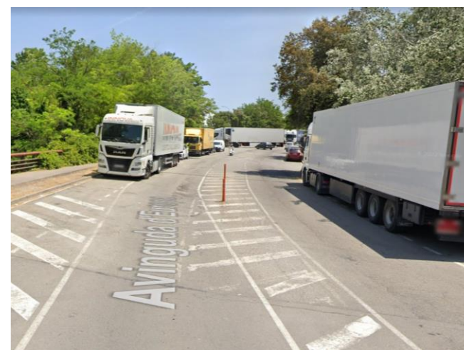
Fissures, trencaments, desprendiments i deformacions.
